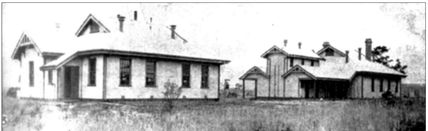
Laundry and bathrooms (left) and disinfecting chambers (right) at the Quarantine Hospital, Coode Island.
