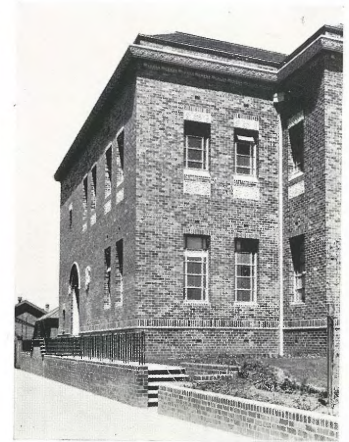
The view, from Hyde Street, shows the entrance to the public assembly hall.
